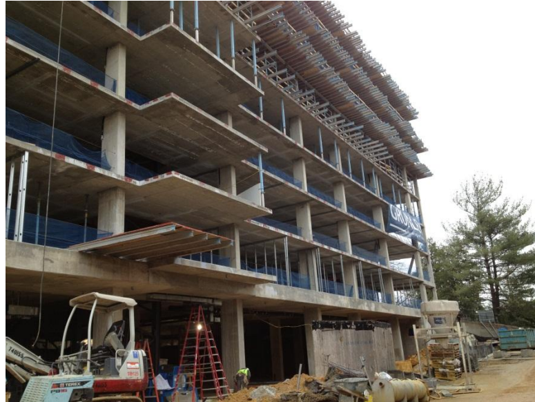
Figure 1: North Hall South Façade
